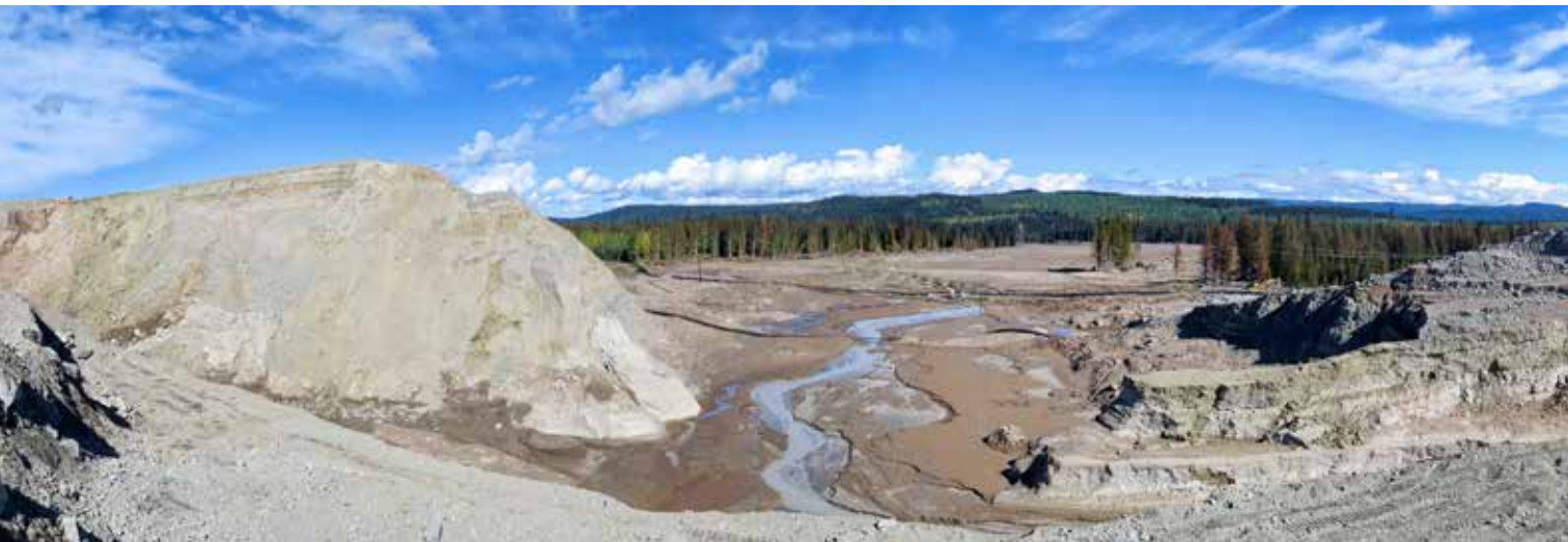
Mt. Polley dam failure. (Top Photo: Reuters.)
