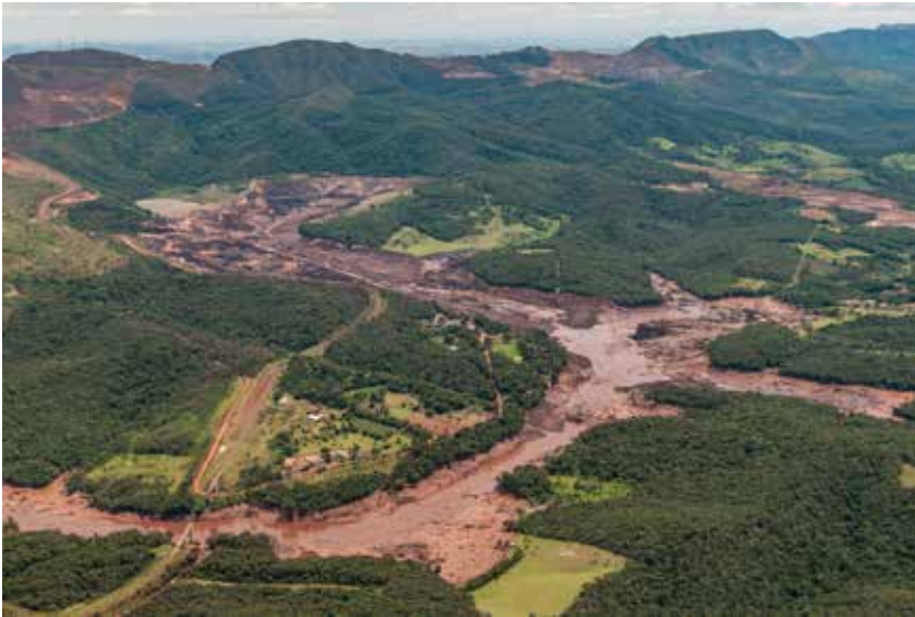
Figure 4. Brumadinho Dam failure. (Photo: Wikipedia.)
